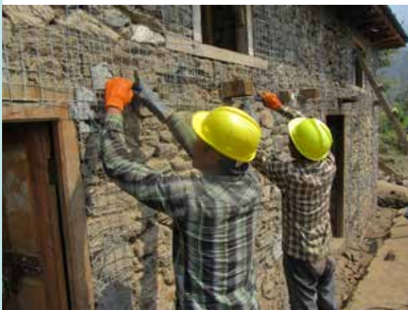
a. Masons Receiving Hands-On Training on Retrofitting
