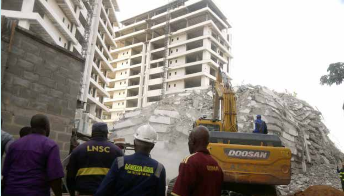
Figure B3.2.1 // Building Collapse in Lagos, 2021
